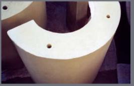
Column sections are aligned with pre-cast holes and pins.
