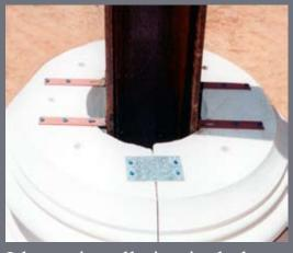
I-beam installation includes L-clips and Tap-Con screws.
